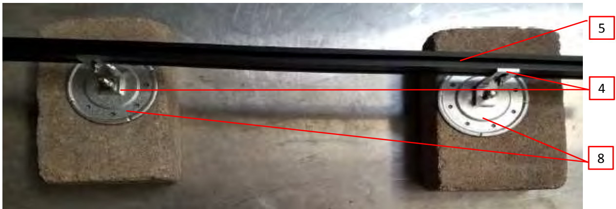
Photo 9- Mechanical anchor Rail and U-Anchor 2600
